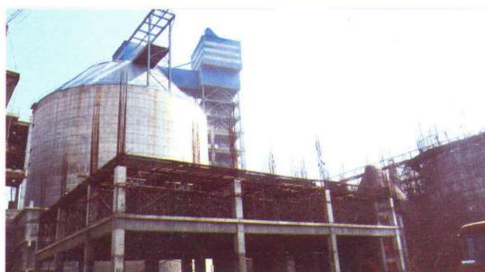
A partial view of Ongoing Expansion project (Unit-III)
